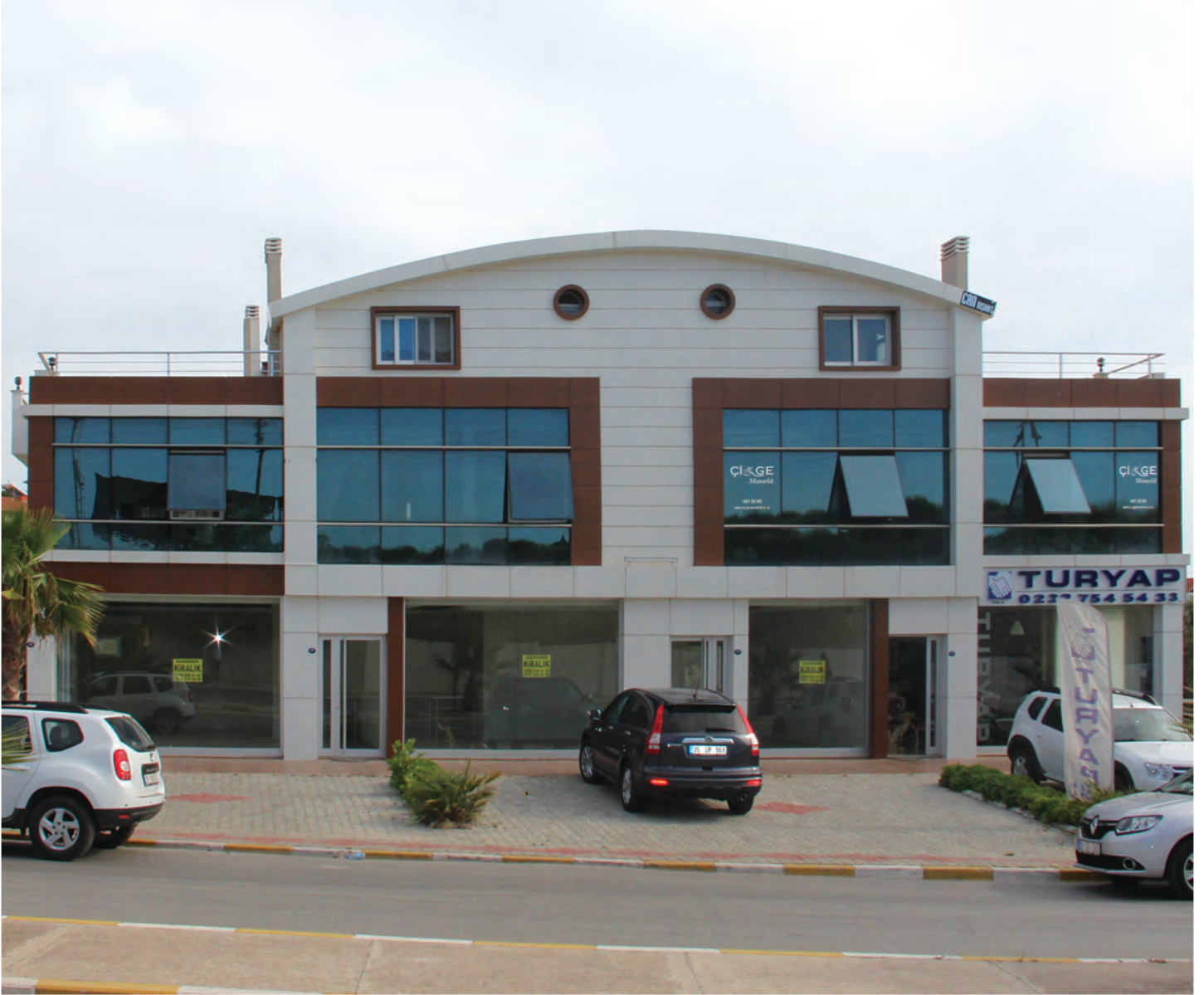
Can İnşaat | Urla
